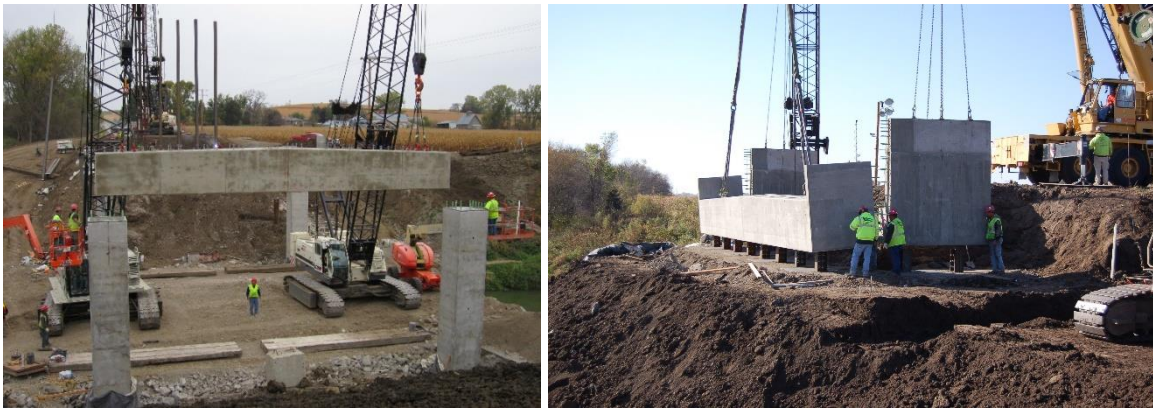
Figure 1.6 Precast substructure in the US 6 Bridge over Keg Creek, Iowa
