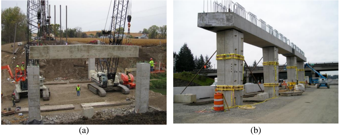
Figure 2.2 Precast frame piers for (a) U.S. 6 Bridge over Keg Creek and (b) U.S. 12 Bridge over I-5 at Grand Mound
