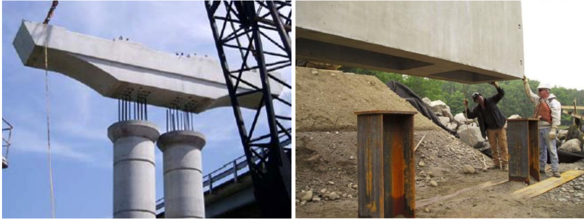
Figure 1.4 Precast bent cap (Lake Belton Bridge, Texas) and precast abutment (Davis Narrows Bridge, Maine)
