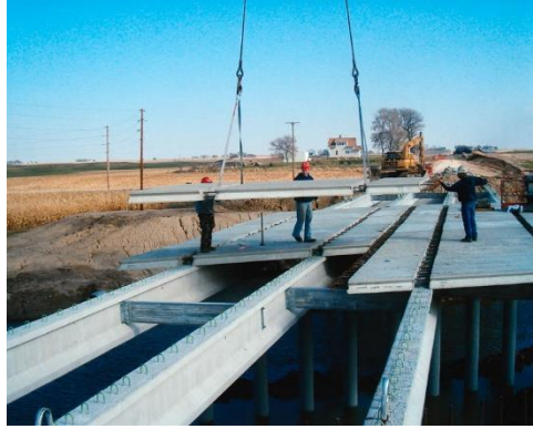
Figure 1.5 Full precast superstructure utilizing precast deck in the Mackey Bridge, Iowa
