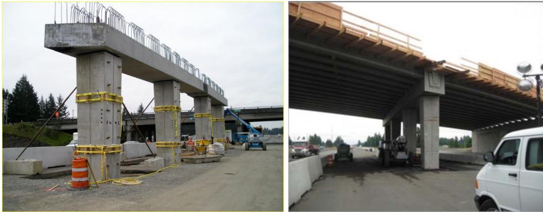
Figure 1.7 Precast substructure and superstructure in the I-5 Grand Mound Bridge, Washington
