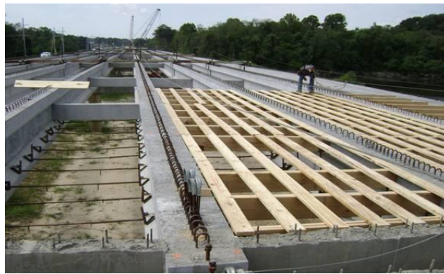
Figure 1.3 Precast girders made composite with deck in the Magnolia Bridge, Louisiana
